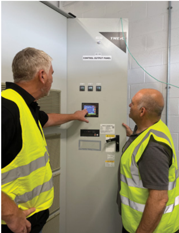
Operating data is visualized in a user-friendly way via the GOT operator terminal from Mitsubishi Electric. Source: Mitsubishi Electric Europe B.V.
